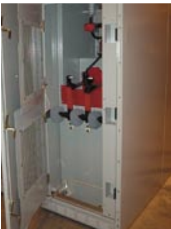
Carrier Dome switchgear: (left) Cable-entrance section; (center) custom-designed bus transition section; and (right) protective relay and control section
