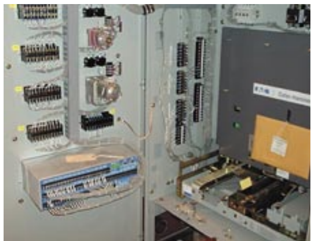
Carrier Dome switchgear: (left) Cable-entrance section; (center) custom-designed bus transition section; and (right) protective relay and control section
